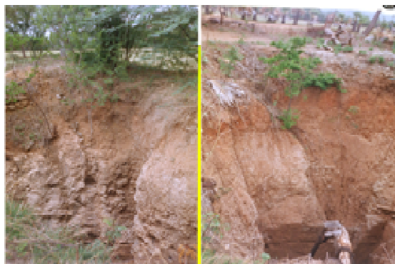
Plate 1 Exposed abandoned well near Ves-station M-3.
